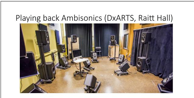
Room 117 uses 24 full-range speakers and 4 subwoofers for full height spatial sound reproduction. There is a routing decoding system to care of patching, ambisonic decoding, speaker balancing and room correction, and the crossovers for distributing sound to the subs. You can send a B-format signal to various decoders or address each speaker individually, depending on settings.
